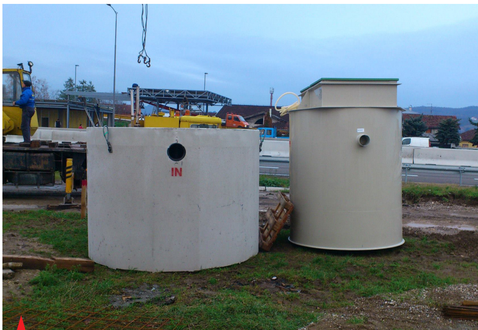
ACO Oleopator petrol and light mineral oil separator (on the left) and ACO Clara Wastewater Treatment Plant
